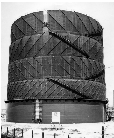
Figure 5: Milan-Bovisa: Telescopic/ 4-lift gasholder, spiral-guided, building year: 1956, capacity: 130.000m 3 . The gasholder was demolished in 2002 (Photo: Archivio Storico Aem, Milan).
