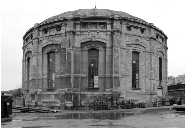
Figure 4: Trieste, Broletto: Telescopic/ 2-lift gasholder, guide-framed with an architectonical ornate gasholder house, building year: 1901, capacity: 20.000m 3 (Photo: Berger 2014).
