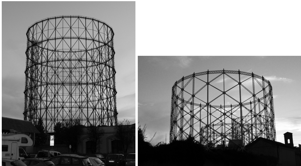
Figure 3a (left): Rome, San Paolo: Telescopic/ 5-lift gasholder, guide-framed, patent of: August Klönne, Dortmund, building year: 1936, capacity: 200.000m 3 . This in Rome called gazometro is one of the tallest remaining gasholders in Italy (Photo: Berger 2013).
