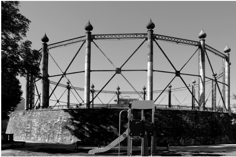
Figure 2: Florence, San Frediano: Bell-type gasholder, column-guided with an ornate ending “flame” on top of the columns, building year: 1882, erected by: V-Ve-Moussy-Constructeur-Lyon, capacity: 8.000m 3 . This was one of the smallest gasholders in Italy. In the 1955 this gasholder got a second so-called flying lift and augmented its capacity to 14.000m 3 . See the following chapter (Photo: Berger 2013).
