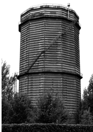
Figure 5: Brescia: MAN Piston-type gasholder, building year: 1947, capacity: 15.000m 3 - the previous identical gasholder was built in 1932 and destroyed in the world war (Photo: Berger 2013). The first dry-sealed gasholder in Italy was built in 1930 in Bologna; patented: MAN Piston-type gasholder, capacity: 30.000m 3 .
